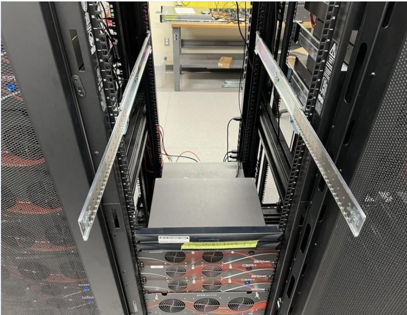
Figure 20: Sliding the unit into the rack.
