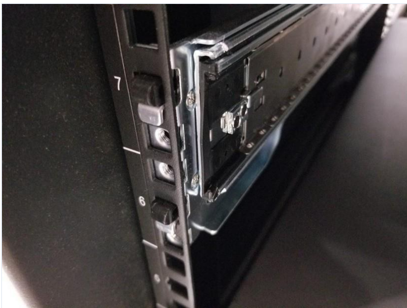
Figure 18: Rails extended, ready for the unit.
